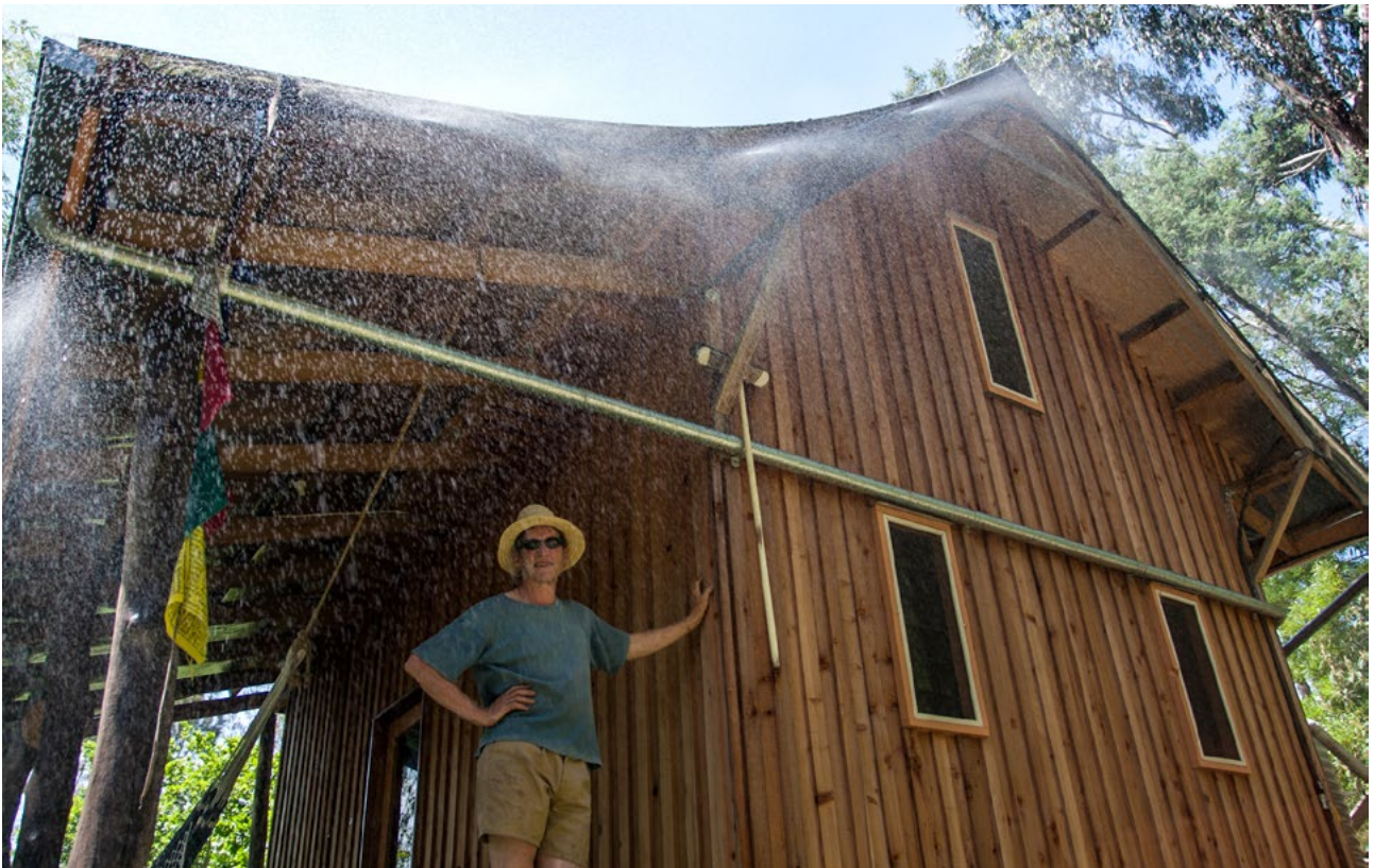
Roof spray systems for more at risk buildings and places, Melliodora 'Tea House'.
